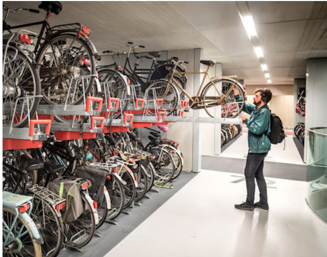
Figure 4.7 - Double-stacked gas-assist bicycle racks
